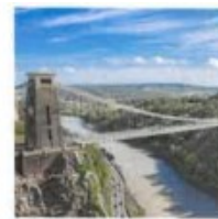
Clifton Suspension Bridge
